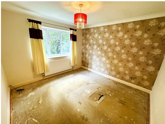
UPVC double glazed window to the rear elevation, central heating radiator and television point.
