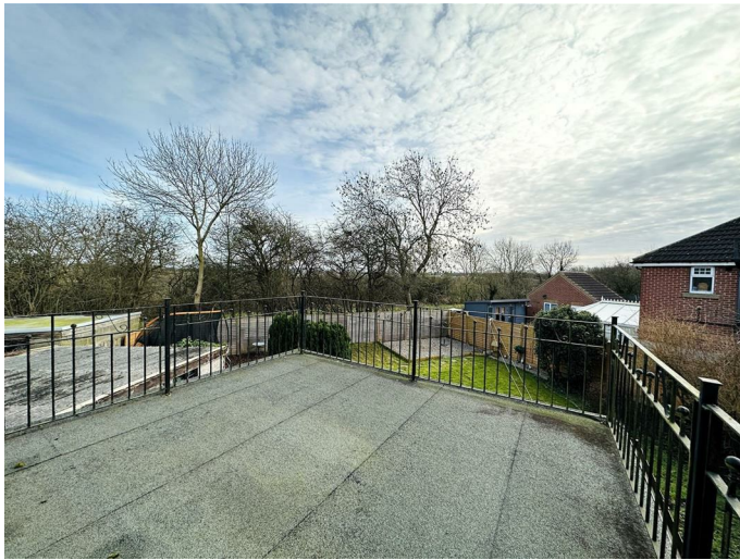
UPVC double glazed window to the side elevation. UPVC double glazed 'French' doors to the rear elevation leading out onto roof terrace with decorative railing. Door leading into:
