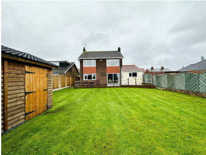
Garden is laid to lawn and fully enclosed with timber fence, concrete posts, decorative gravel boards and brick wall.
