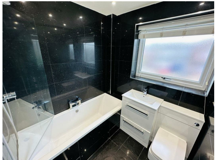
White bath with chrome mixer tap over and chrome shower with chrome controls. Glass shower screen and tiled side. White low flush w.c with concealed cistern and chrome controls. White wash hand basin with chrome mixer tap over set into white high gloss vanity unit with chrome 'T-bar' handles. Chrome heated towel rail, extractor fan and tiled flooring. The room is tiled on all walls to ceiling height. UPVC double glazed frosted window to the front elevation.
